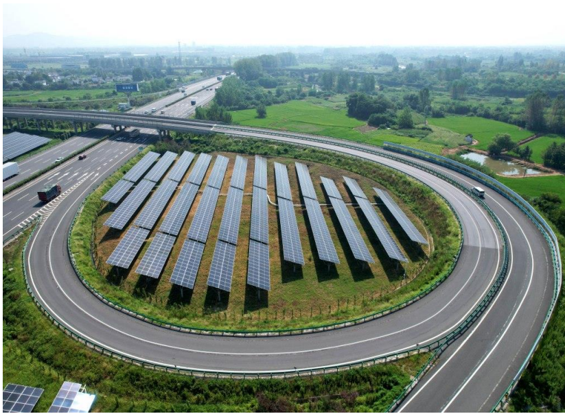
Sub-belt photovoltaic power station installed in the G5011 Wuhu-Hefei Expressway test tunnel in Chaohu, China. Costfoto/NurPhoto/Shutterstock
